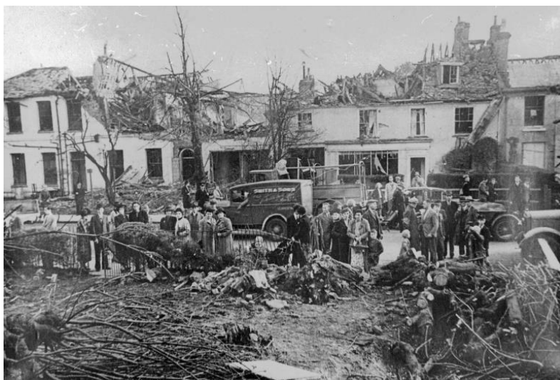
World War Two bomb damage in Bells Hill (above) and Wood Street
