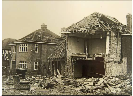
Photograph: Bomb damage in the Hadley Wood area
