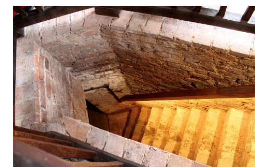
Photograph: Stairs leading to the Sumps
