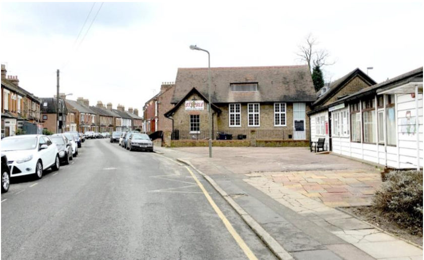
Salisbury Road 2019. The Fern Rooms (on the right) were demolished in 2020
