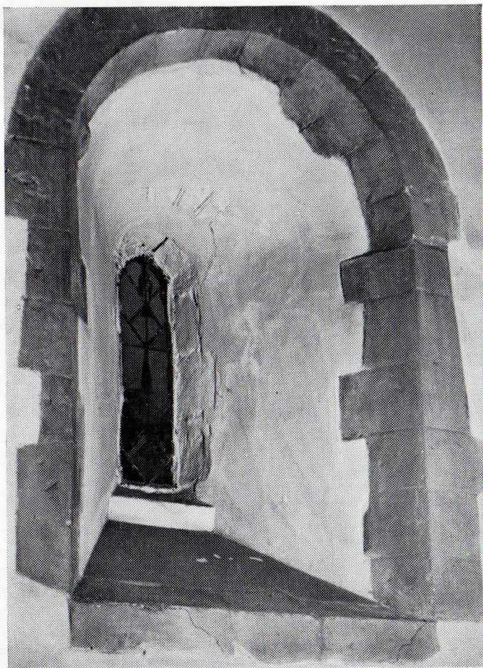
ONE OF THE WINDOWS IN THE NORTH WALL
