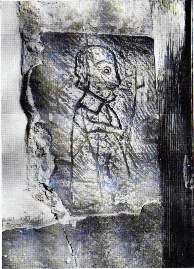
A DRAWING ON THE WEST JAMB OF THE INNER DOORWAY OF THE SOUTH PORCH
